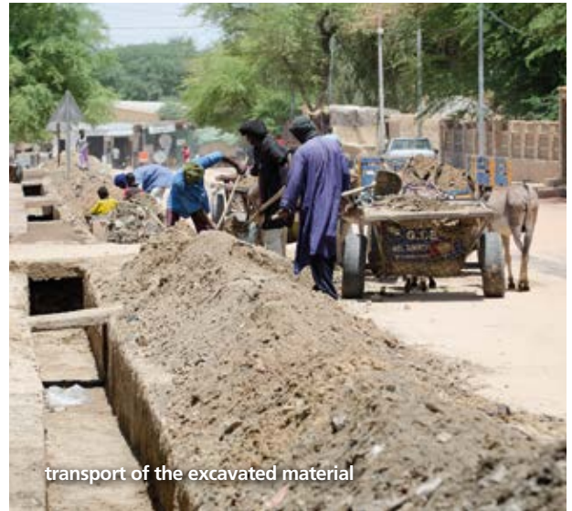
The storm water channel in Timbuktu is being cleaned from sand and waste.
