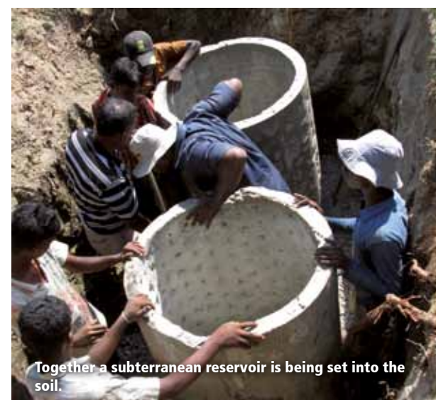
The fundament of the water tanks and filters of the water treatment plant is being built.
